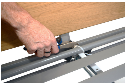
You may now remove the transportation safety ties from the mattress base by cutting through the cable ties with a side cutter or a knife.
